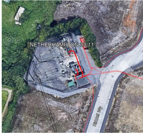
Figure 15 Aerial view of Netherhampton PSS
