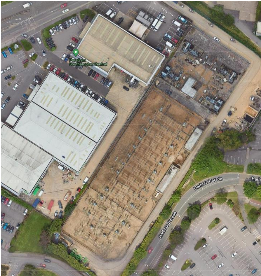
Figure 2: Southampton BSP aerial view
