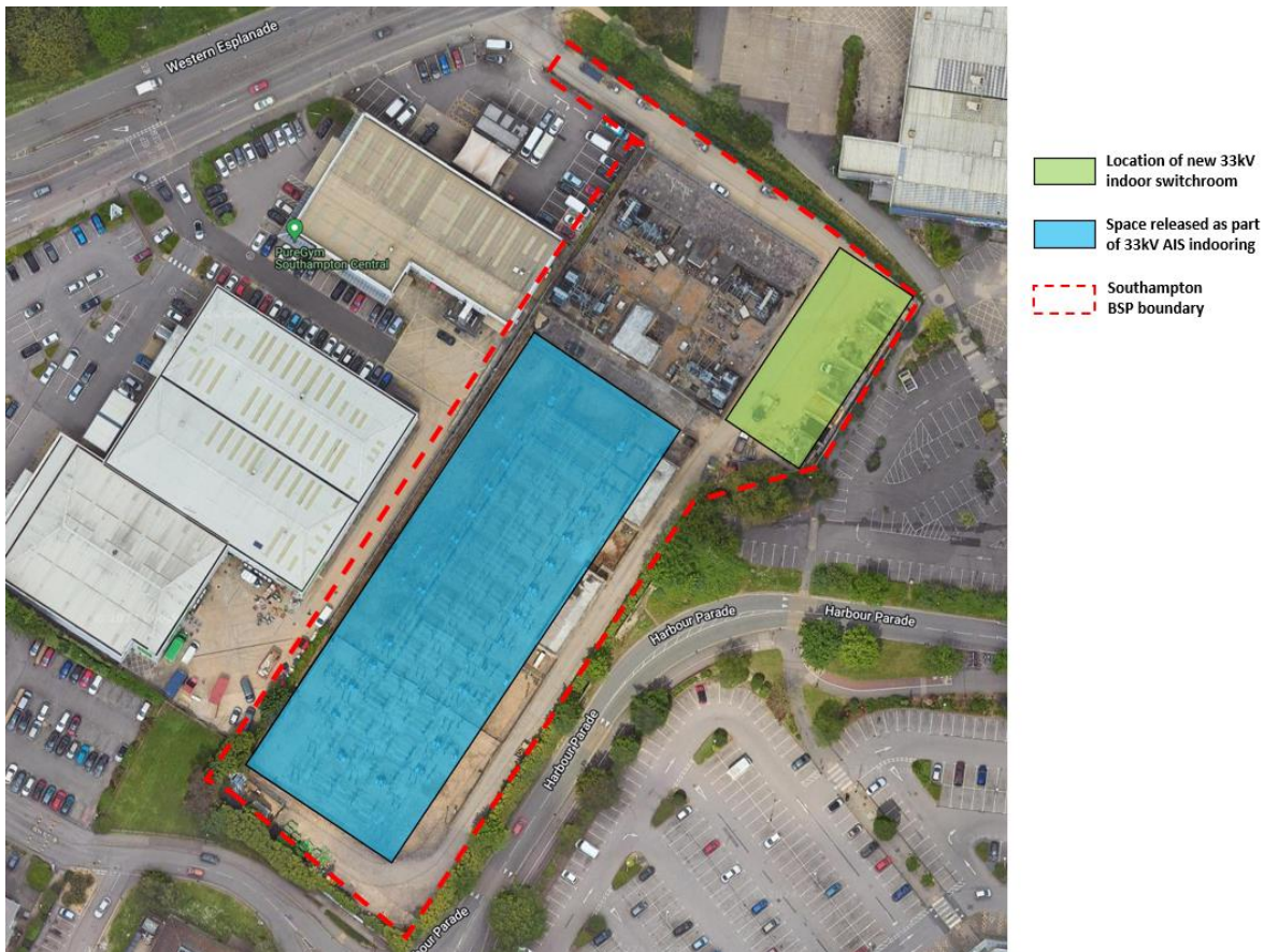
Figure 10: Aerial view of Southampton BSP, with the location of the new 33kV indoor switch room and subsequent space released
